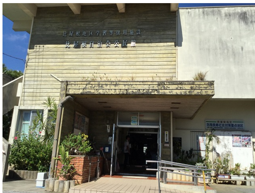
図2 Hineya community center
